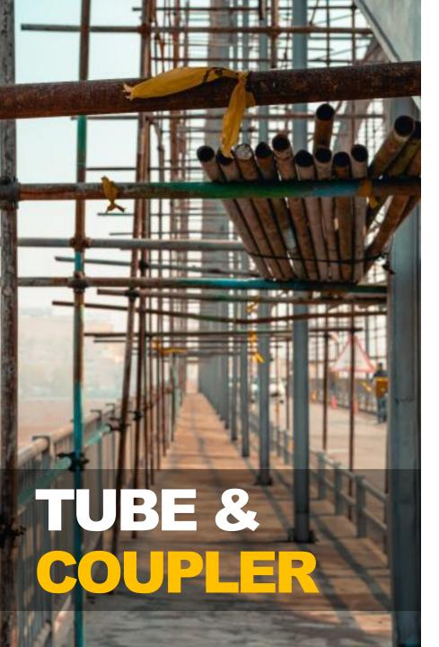
One of the most common types of scaffolding used in construction purposes.
