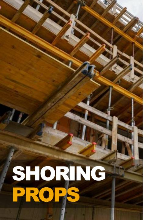
Telescopic steel props with flat plates fitted to the outer ends, and a robust nut and pin arrangement in the middle for length adjustment.
